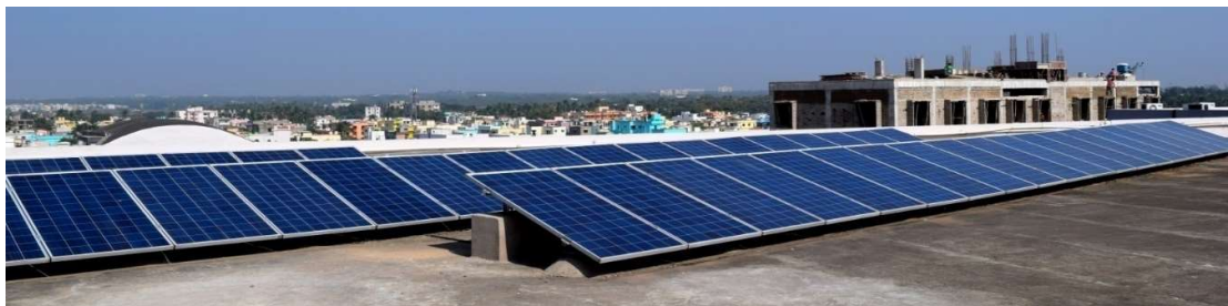
Fig. 2: Setup of rooftop-based 11.2 kW PV system at Siksha 'O' Anusandhan Bhubaneswar Campus.
